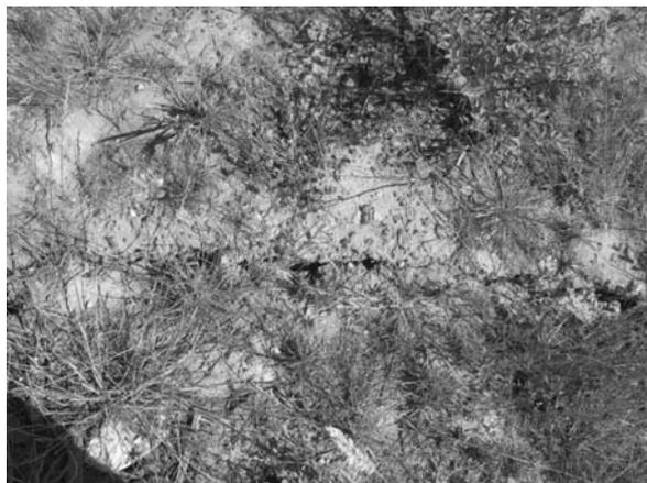
Fig. 1.3. Fissure in soil at place adjacent to roadway A4 from North (Wirek parking place)
