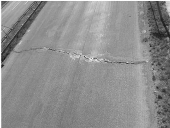
Fig. 1.1. Discontinuity on southern roadway of A-4 – direction Kraków
