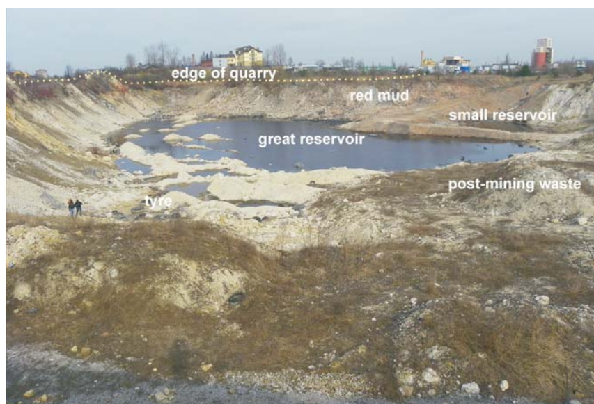
Fig. 4. View of the Górka reservoir after pumping of leachate (photo by E. Pietrzyk-Sokulska)
